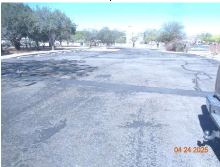
Asphalt - cracks/damage noted - recommend review, possible total replacement
