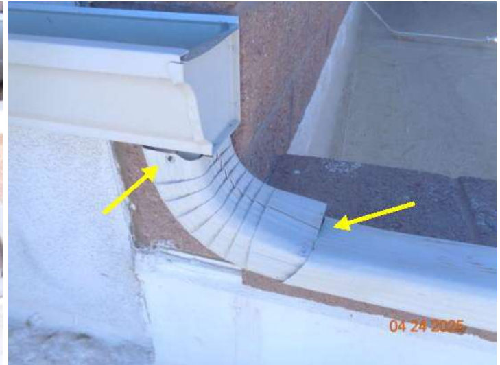
loose/damaged/disconnected
