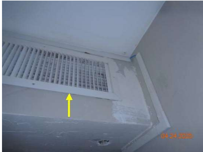
missing screws - vibrates
