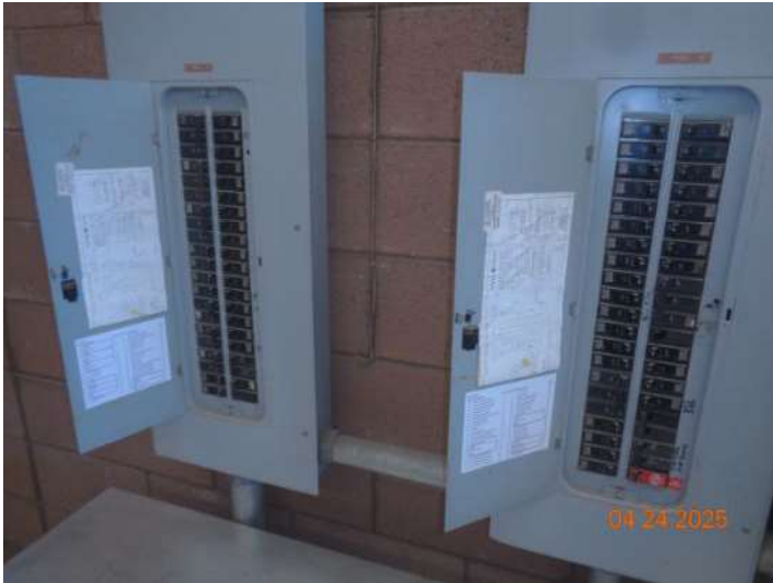
Panel Does Not Have Proper Clearance
