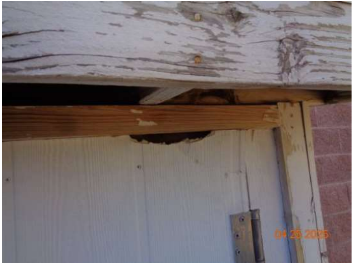
sheds not inspected: noticed weathered /damaged wood
