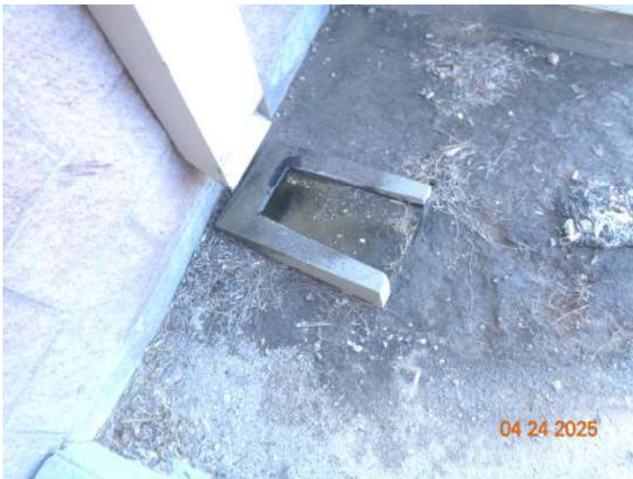
does not divert water away from structure
