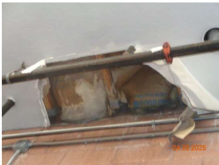
drywall open - seller stated from past roof leak
