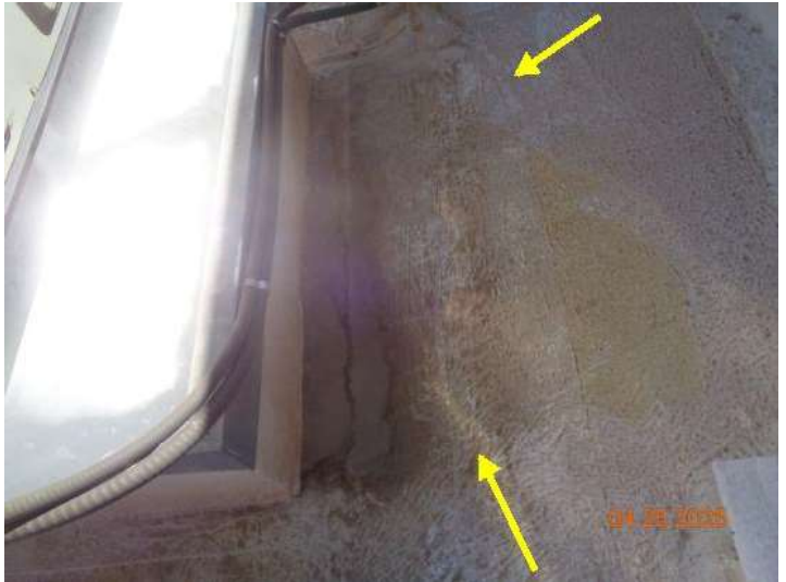
Elastomeric touch up is needed on various areas.
