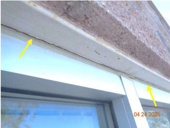
Some exterior frames need to be caulked.
