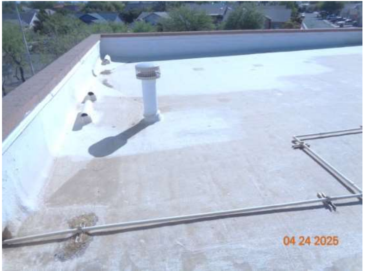
Elastomeric touch up is needed on various areas.
