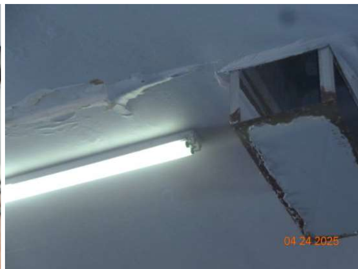
evidence of past leaking
