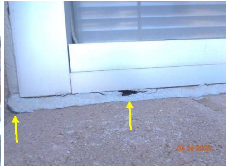
Some exterior frames need to be caulked.
