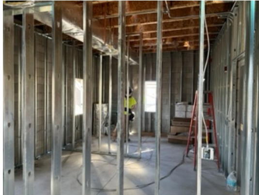
Turnout/decon interior framing walls
