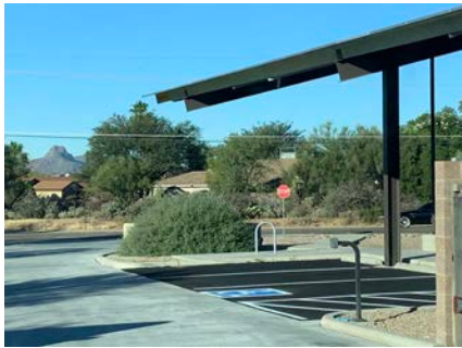
Station 379 : concrete and asphalt
